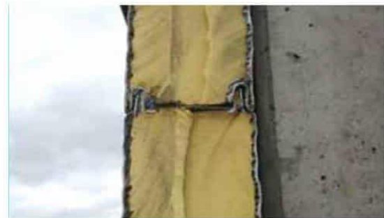
Picture 33. View of burnt panel cut with an angle grinder.
