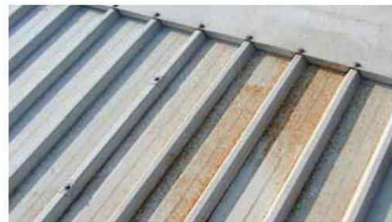
Picture 34. View of lacquer coating damaged by filings during cutting with an angle grinder
