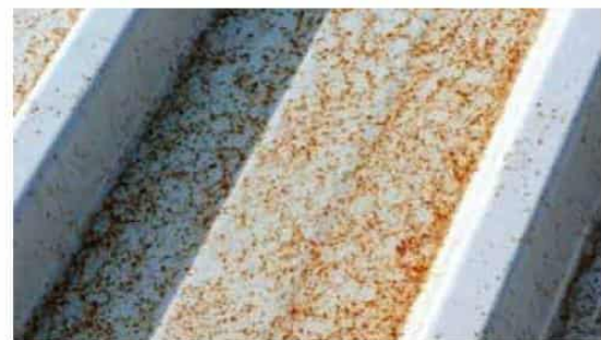
Picture 35. Damage to lacquer coating caused by leftover rusted filings
